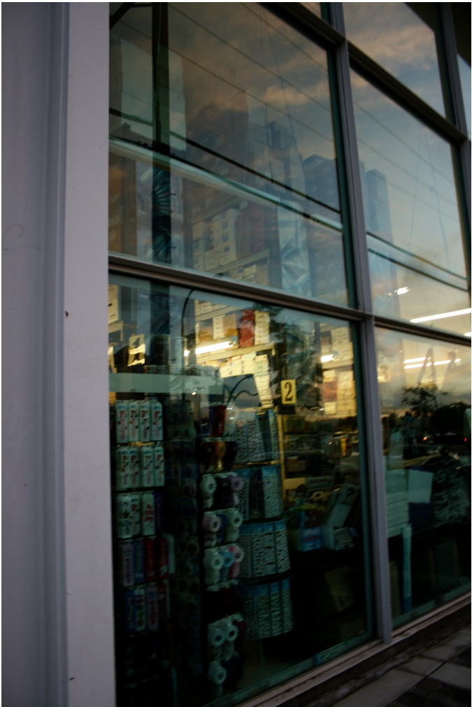
Suspected hazardous fire conditions
